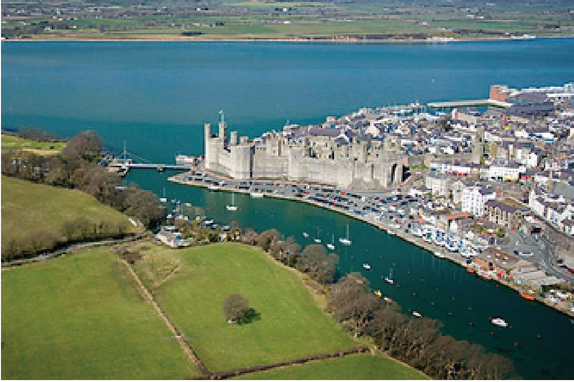
Figure 1.27 Contemporary photograph, aerial View of Caernarvon Castle.
